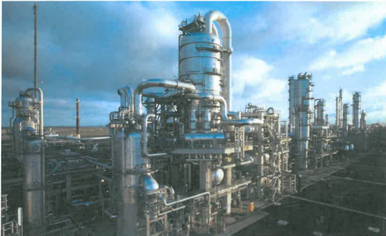
LyondellBasell's Maasvlakte, Netherlands, plant is one of three facilities that the company operates in the Rotterdam port area. It is the largest propylene oxide (PO)/styrene monomer (SM) plant in the world where PO and SM are produced based on the company's unique PO/SM technology. Source: LyondellBasell
